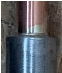
Copper to steel brazed joint.
