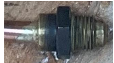
Copper to brass brazed joint.
